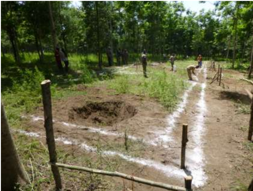
School foundations marked out
