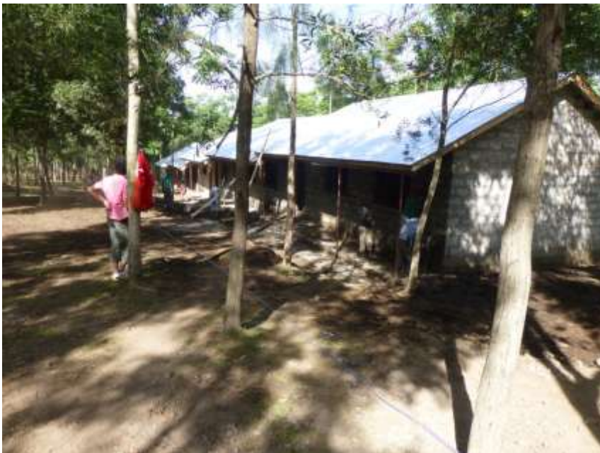
School almost ready
