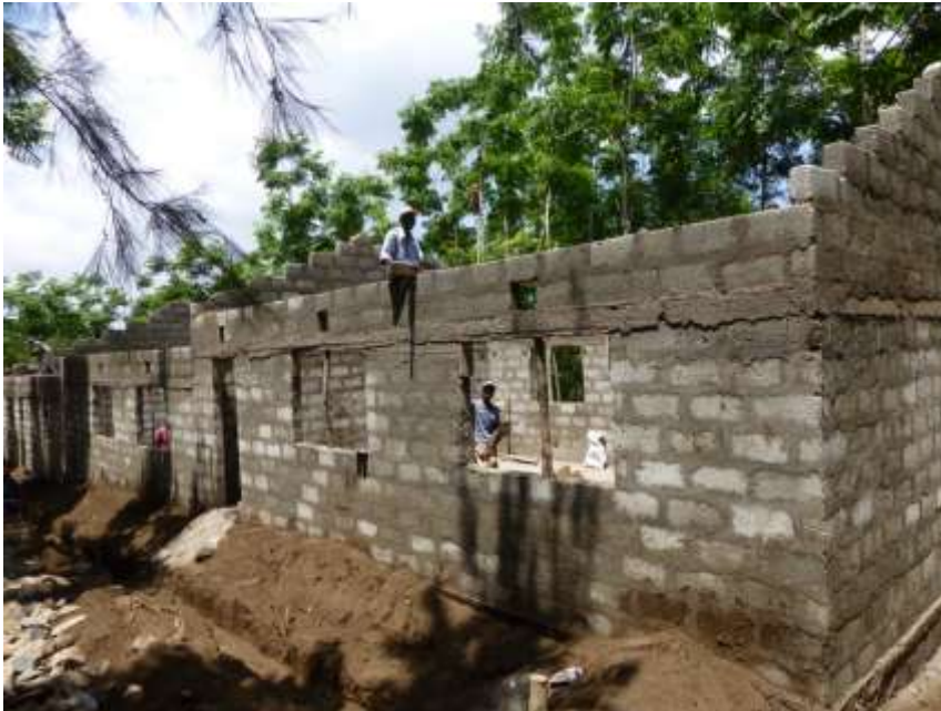
Starting School roof
