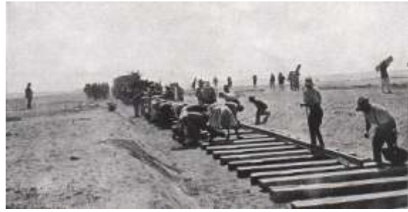
Laying tracks across the Sinai Desert
